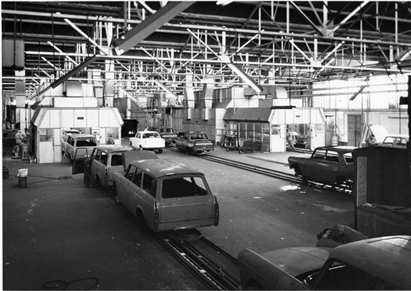
USINES RAGHENO- PAINT SHOP
