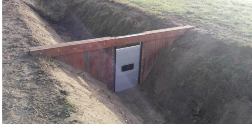
Stuw in “damwand” (bron K.W.T.)
