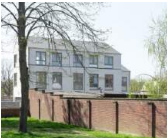
Spoortuin Puurs, Plusoffice architects
