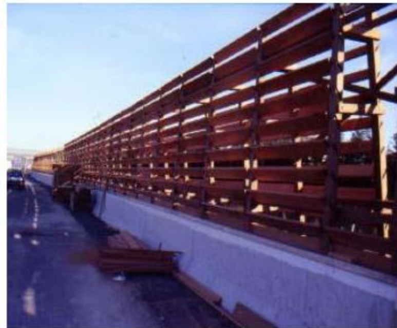
Figure 65 - Bio barrier with wooden structure
