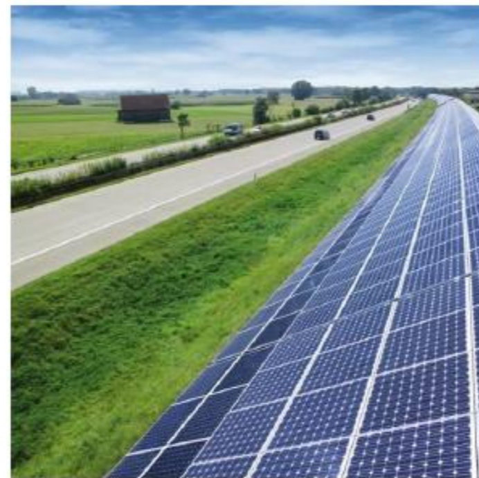
Figure 73: Example of noise barrier with photovoltaic modules
