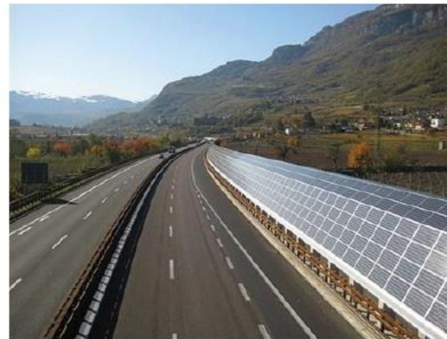
Figure 73: Example of noise barrier with photovoltaic modules
