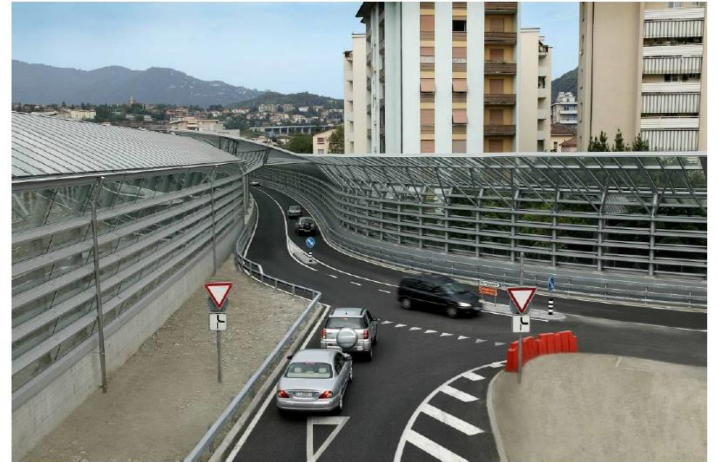
Figure 34: Noise barrier dominating the landscape
