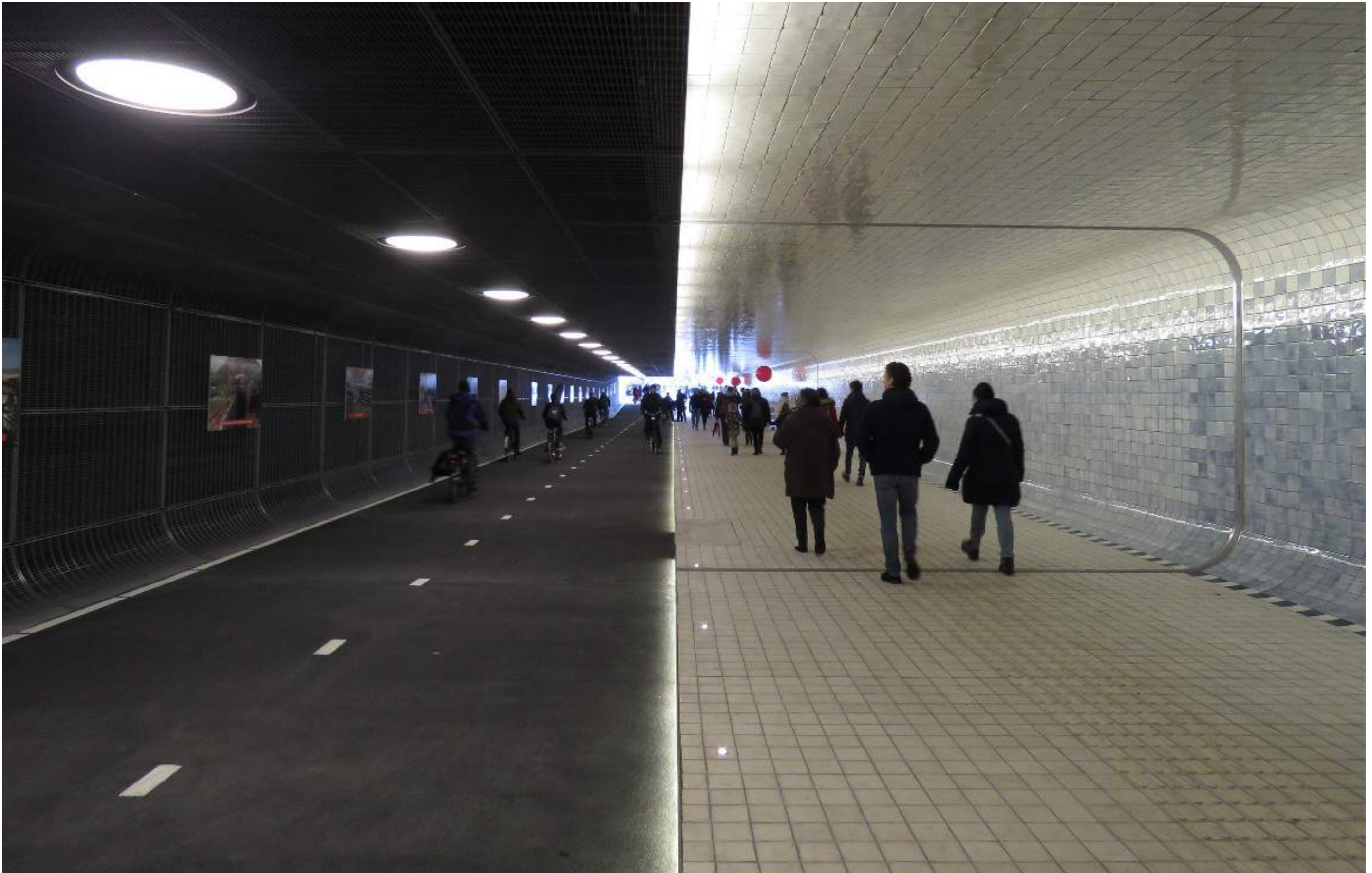
Referentieproject: Cuyperspassage in Amsterdam (Architect: Benthem Crouwel Architects)
